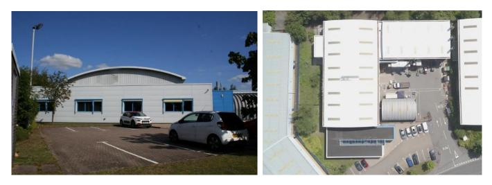
The building in principle is of modern design and construction, being of steel frame with twin skinned cladding and the works area being complete with concrete flooring throughout.
